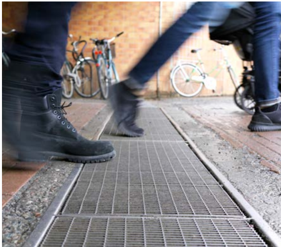
WALKWAY GRATING, STAINLESS STEEL TYPE A
